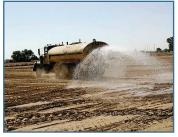
wet soils into workable materials. After spreading the lime, disc harrows alone may be adequate for mixing in extremely wet situations, but rotary mixers are still preferred for heavier soils.
