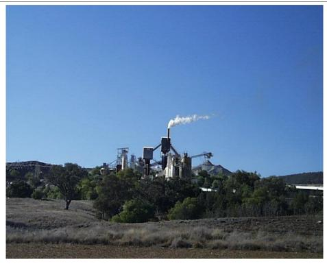
The Attunga Limestone Mine and Manufacturing Plant is located approximately 20Km north-west of Tamworth and 1.2Km northeast of Attunga. Open cut mining operations, using drilling and blasting, produce limestone feed for the processing plant. Two vertical kilns produce lime which is despatched in bagged or bulk form. Crushed rock products are also produced.
