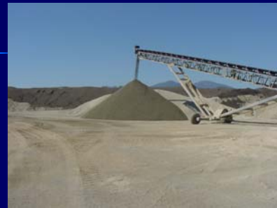
Stacking lime treated aggregate
