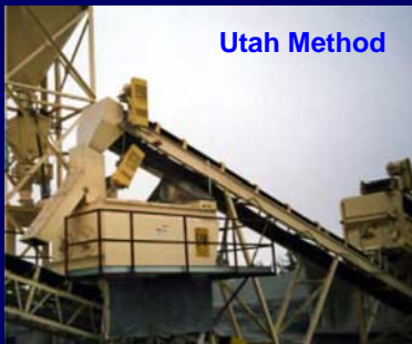
Hydrated lime added to aggregate and fed into pugmill for mixing
