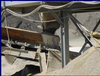
Limed aggregate being discharged from pugmill
